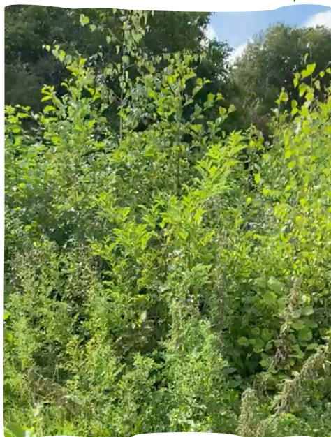
Northern site - Soil excavated to 1m depth
